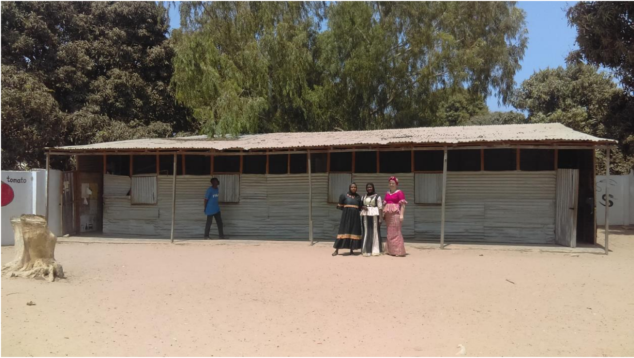
Current school in Batokunku. We have just started construction of a 12 classroom school building here.
