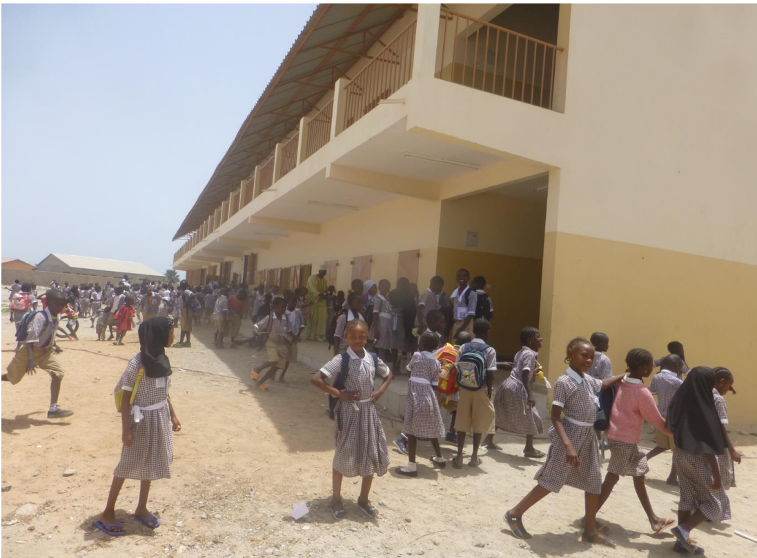
Busumbala Tumbunto Lower basic School. The new building with 12 classrooms + toilets + teacher rooms has been finished recently
