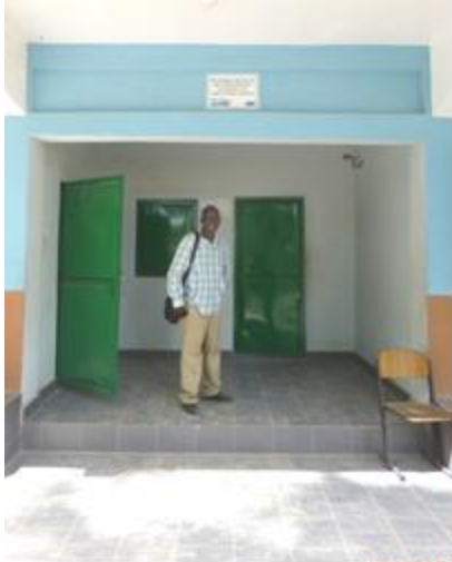
Handing over to the Ministry and school authorities upon completion
