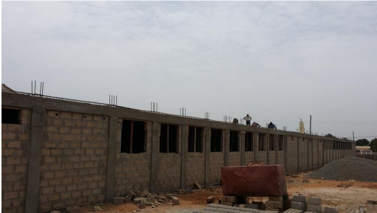
Construction of the new building in Kombo Kerawan
