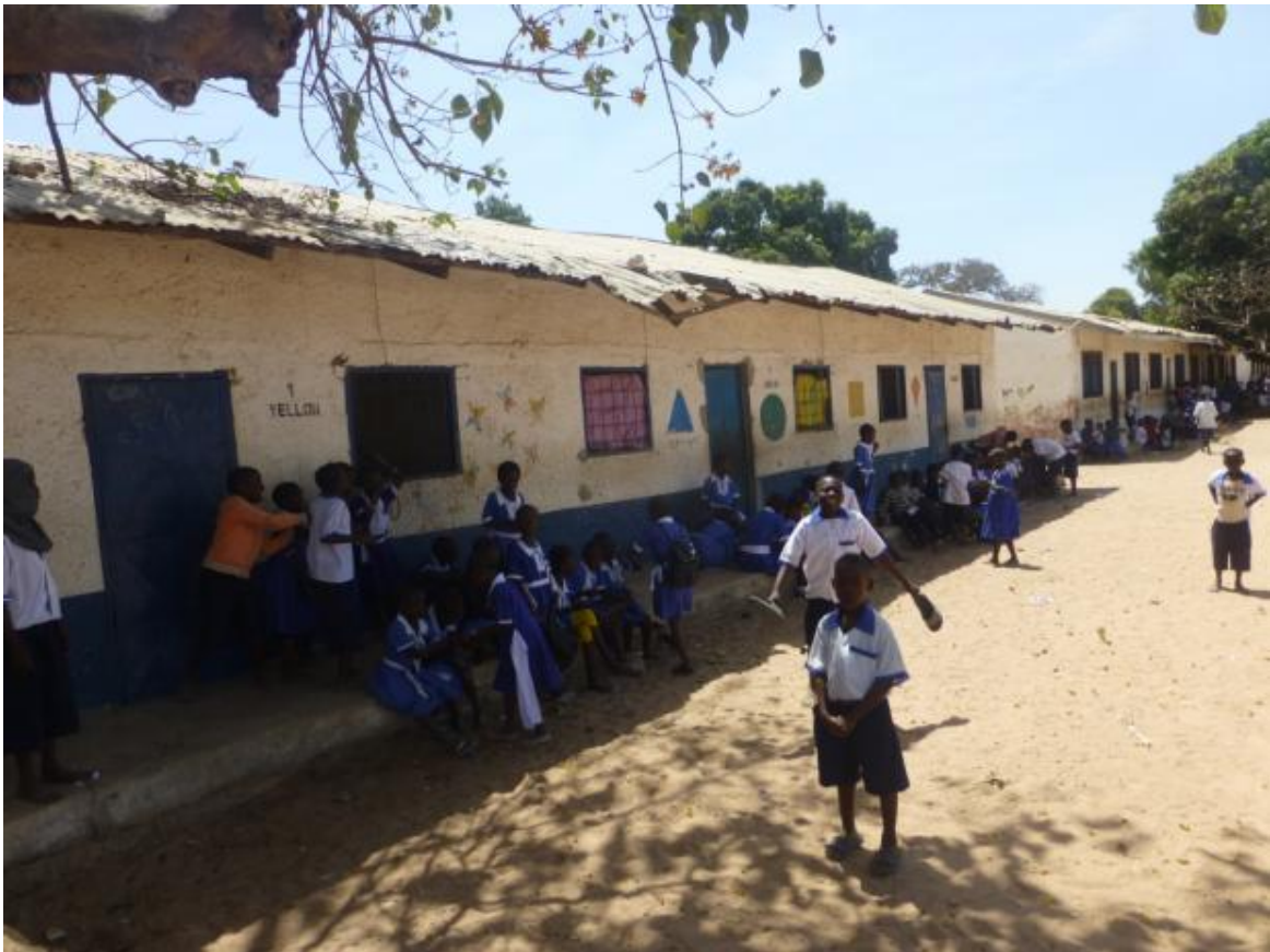
Above: The current Kabafita primary school. This school has 50 class rooms and 3467 pupils! We will build a second school next to the current one. A large project: 30 class rooms.
